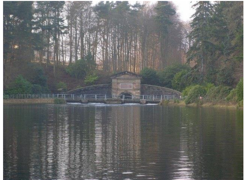
Figure 4.7: Conduit screen wall, Craigmaddie Reservoir
