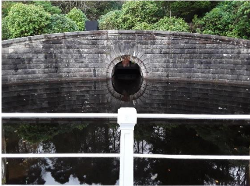
Outlet and gauge basin of Mugdock reservoir
