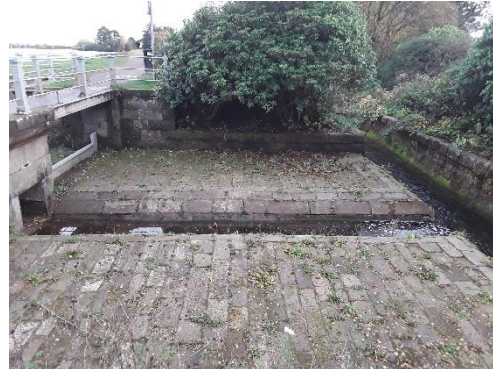
Outlet from Mugdock south dam, rill connecting with Tannoch Loch to the south
