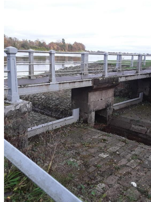
Bridge over overflow channel, Mugdock Reservoir
