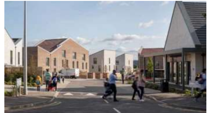
Example of residential use (image c. 7N Architects)
