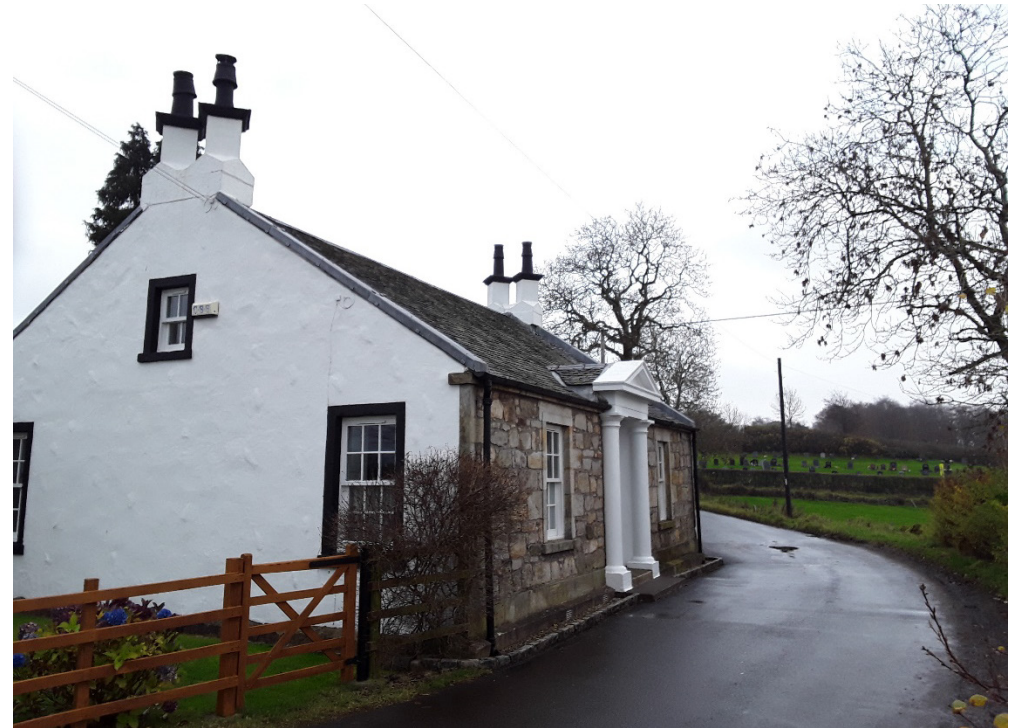
Figure 4.5: Polite architectural detailing
