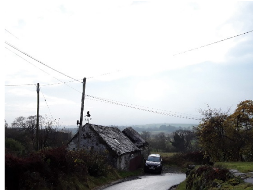
The dilapidated outbuilding on Dowan Road. Note its simple, vernacular appearance, with harled and lime washed elevations, slate roof, low-slung pitched slate roof, linear form, and positioning at the back edge of the road. The silhouette of its weathervane can also be made out.
