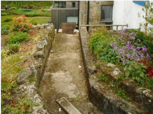
The lade leading up to the water wheel at the old mill.
