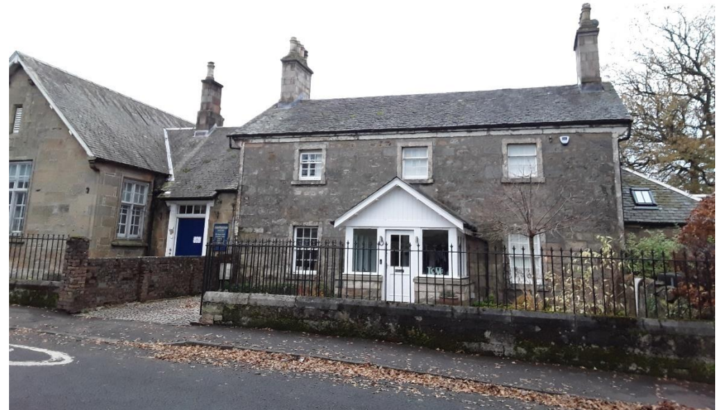
The early-19 th century old schoolhouse with its moulded window surrounds, sash windows, gable end chimneys and coursed and squared stonework. To the left, the gable end of its later 19 th century extension with overhanging eaves and bargeboards.
