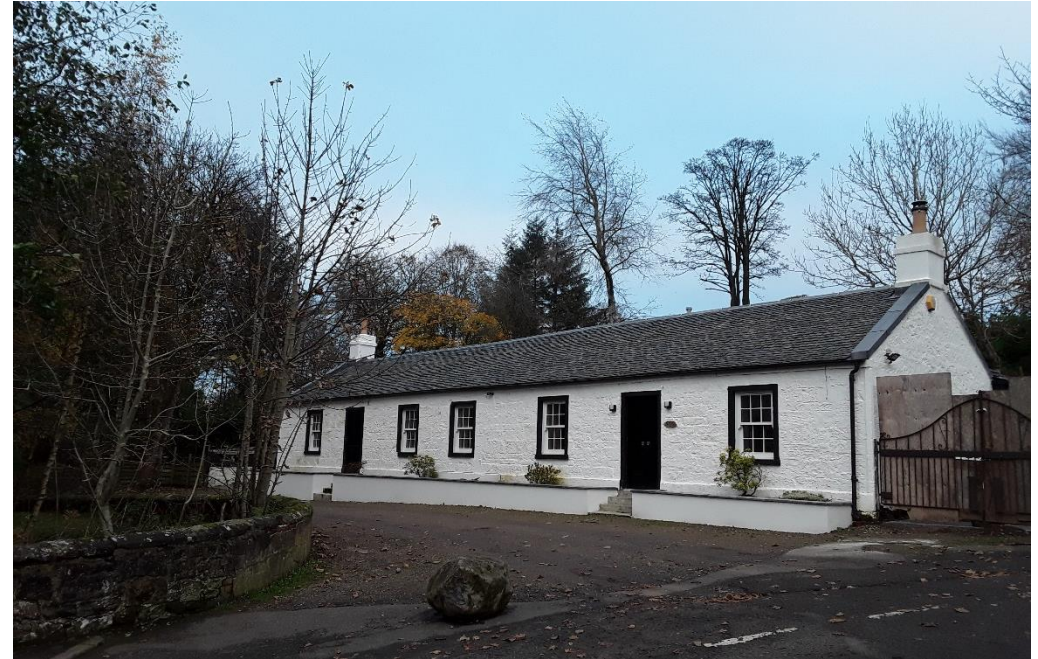
Figure 4.4: The vernacular form of the canal cottages
