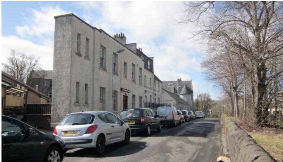
Luggiebank Road looking west
