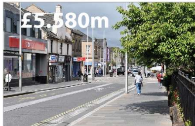
Roads and Footways
