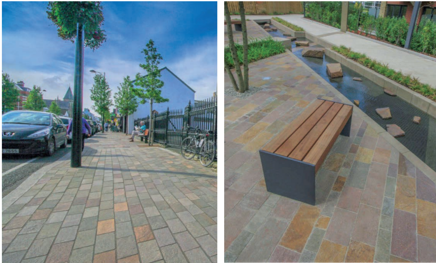
Figure 20: Natural stone porphyry sett and slab paving and in a streetscape
