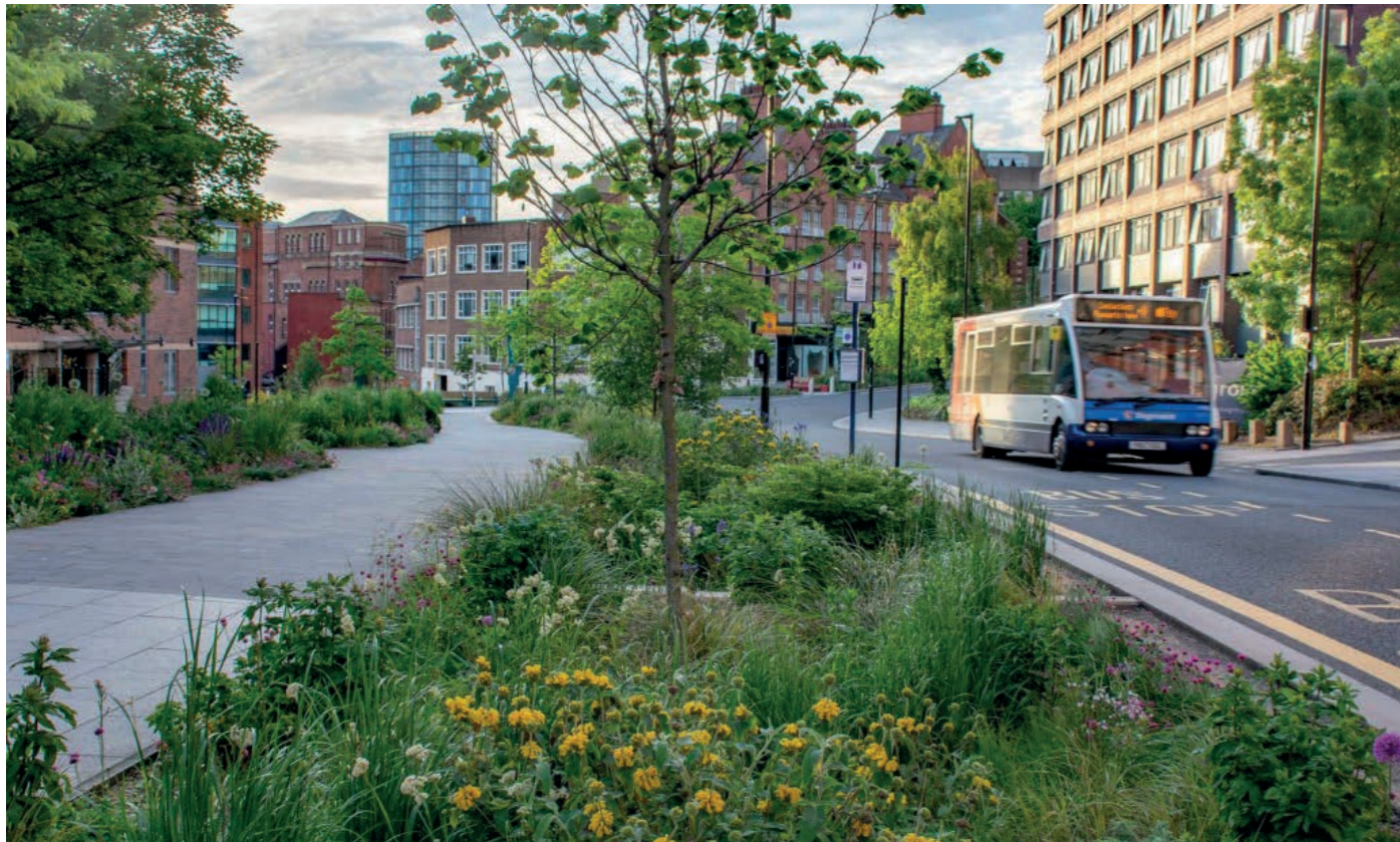
Figure 22: Raingarden SuDS feature, Sheffield
