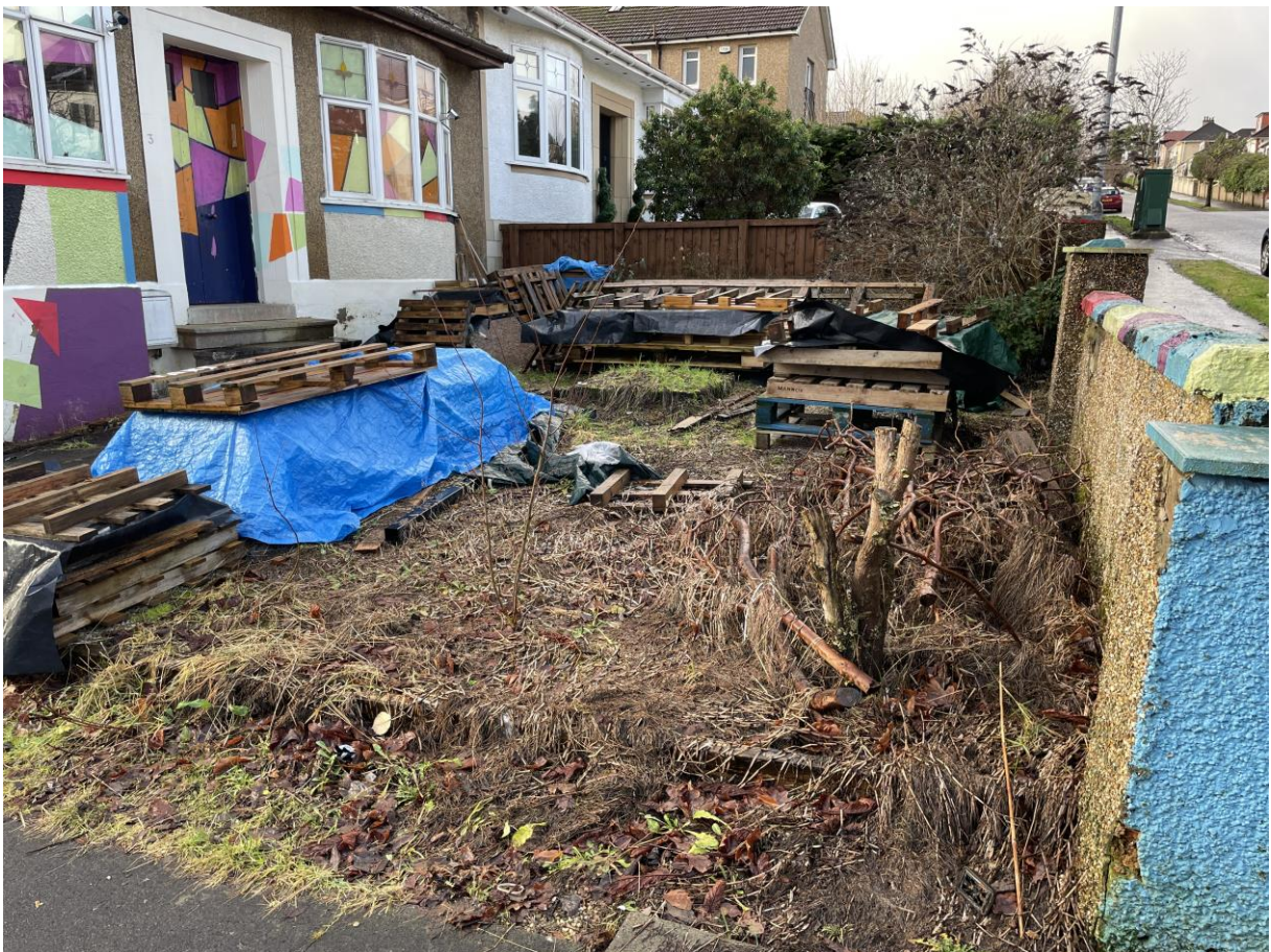
Photograph 1 – Pallets and waste materials in the front garden ground
