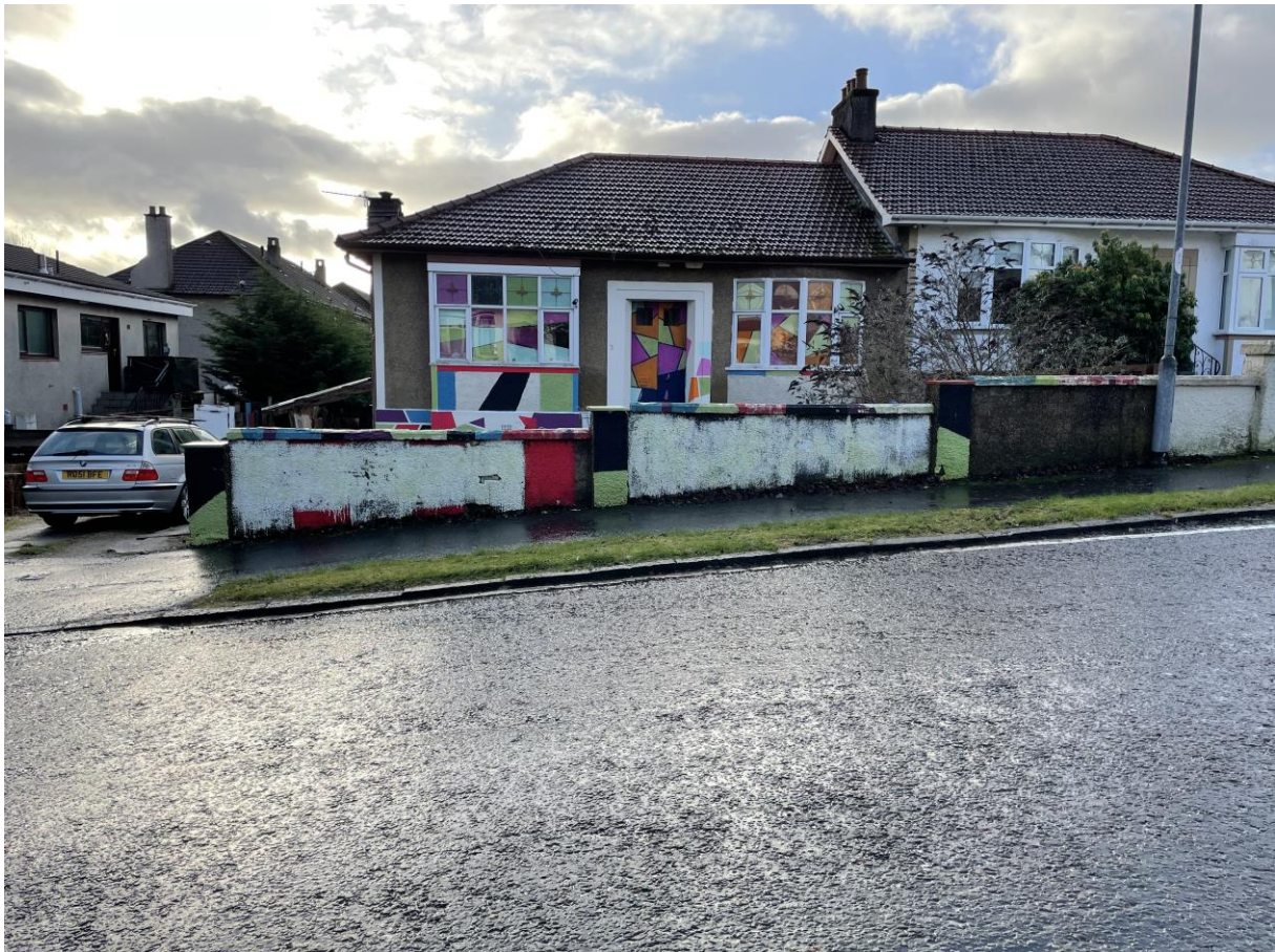
Photograph 3 – Painted front surface of front boundary wall.
