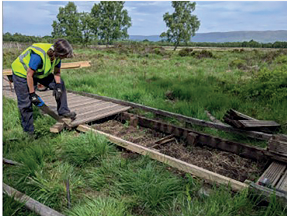
Figure - Green Infrastructure Enhancements, Lenzie Moss
