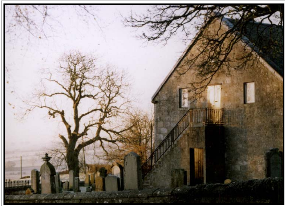
BALDERNOCK PARISH CHURCH
